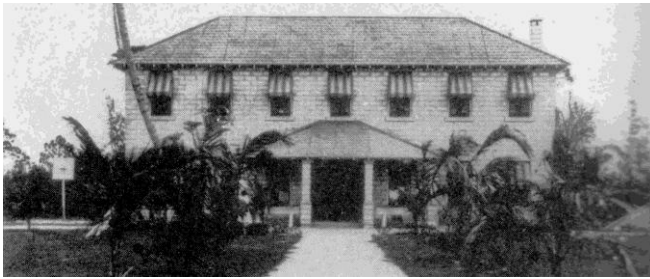
Lantana-Hypoluxo School after it was reopened in 1922 and improved with awnings, trees and playground equipment.
