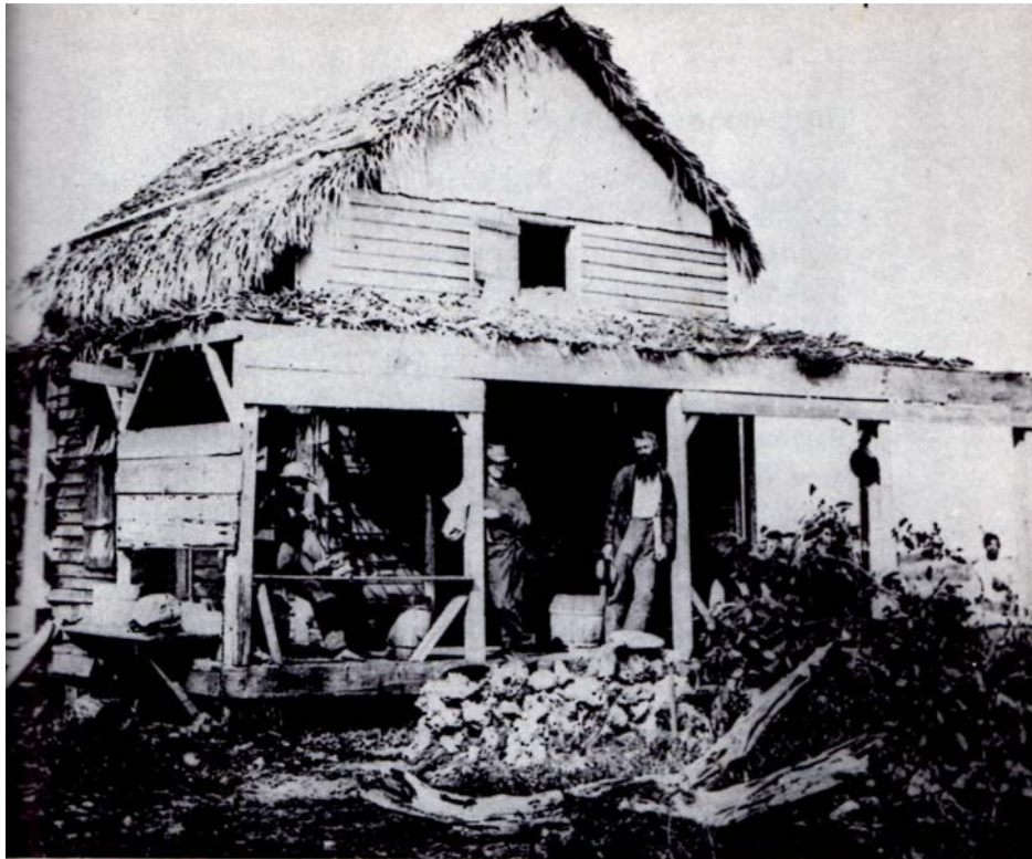
The Pierce home on Hypoluxo Island was built in 1876 from lumber and driftwood salvaged from the beach. H. D. Pierce is leaning against the doorway on the right
