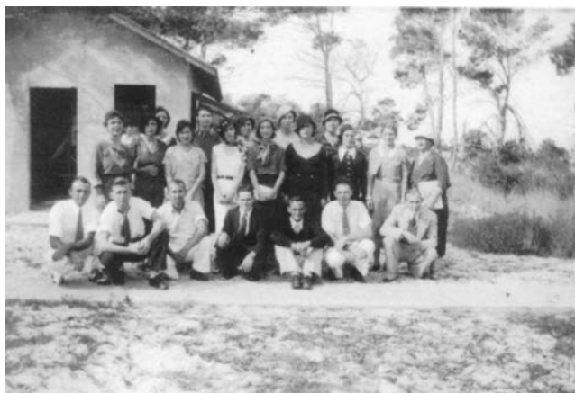
The 1930s Methodist Sunday School building on original site
